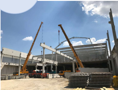
New hall construction
